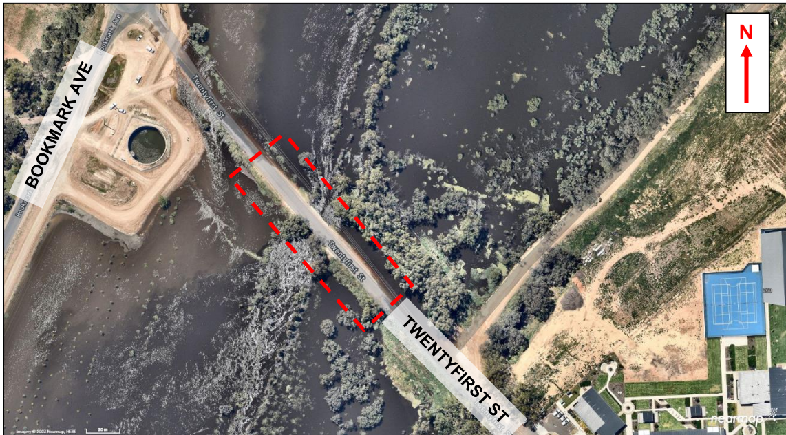
Figure 1 - Aerial image of the site in question, 21 st Street Bridge, Renmark SA (dated November 2022).
