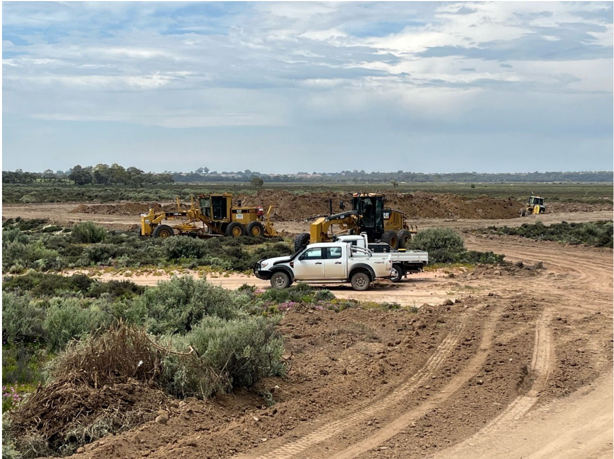
Raising clay to be stockpiled for use on levee remediation
