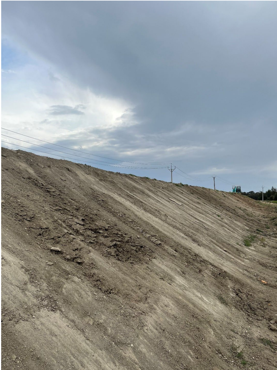
Removing vegetation to prepare the Hospital Levee for remediation works.
