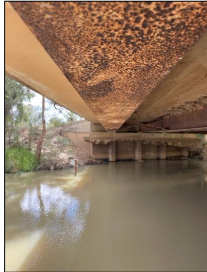
Photo 15 – Steel beam condition indicating minor level of corrosion, no sectional losses.
