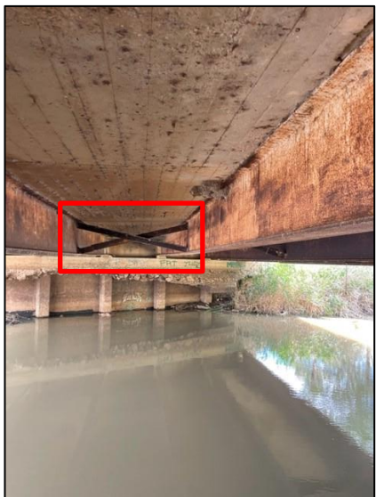
Photo 14 – Steel beam #4 displaying minimal torsion buckling (bottom flange showing minor curvature)
