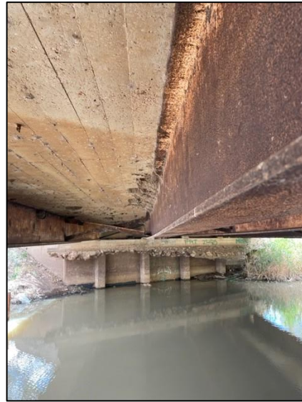
Photo 13 – Steel beam #2 displaying minimal torsion buckling (bottom flange showing minor curvature)
