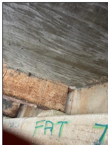
Photo 11 – Prior completed repairs (East end of bridge)
