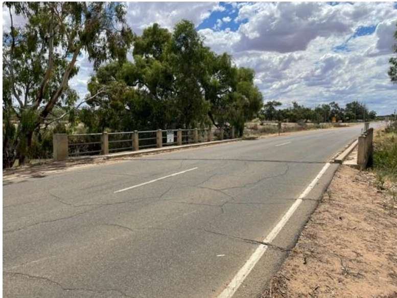
Photo 1 – 21 st Street Bridge, Renmark SA (orientation facing North)
