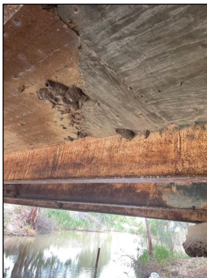
Photo 10 – Prior completed repairs (East end of bridge)
