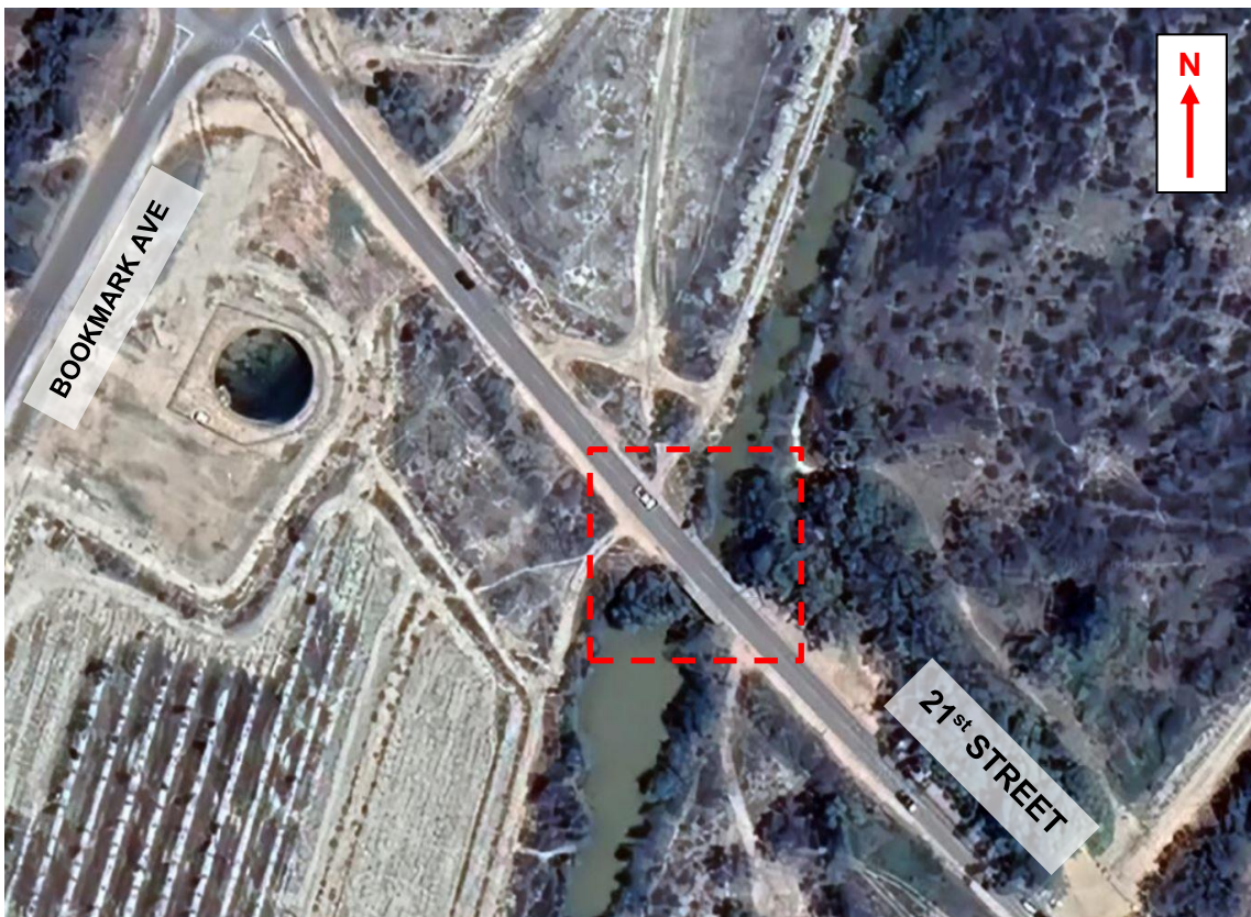
Figure 1 - Aerial image of the site in question, 21 st Street Bridge, Renmark SA (dated February 2022).
