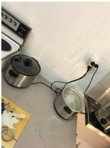
Double adapters used for electrical appliances
